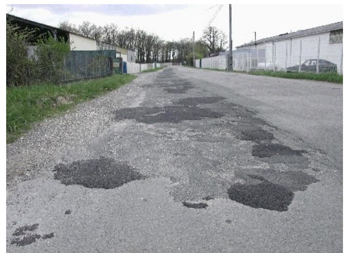
Reprofiling and resurfacing with 2 layers of dense cold mix (0/10 mm).
