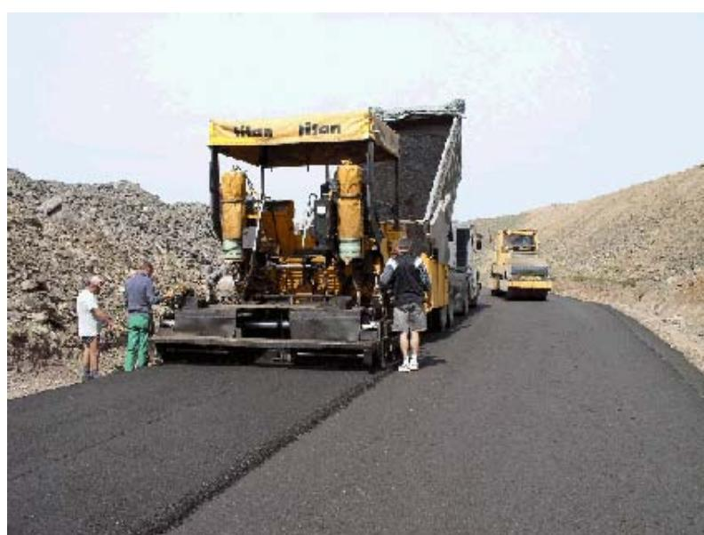
Good resistance to heavy loads traffic (quarry road) despite of high void content (15% after one month).
