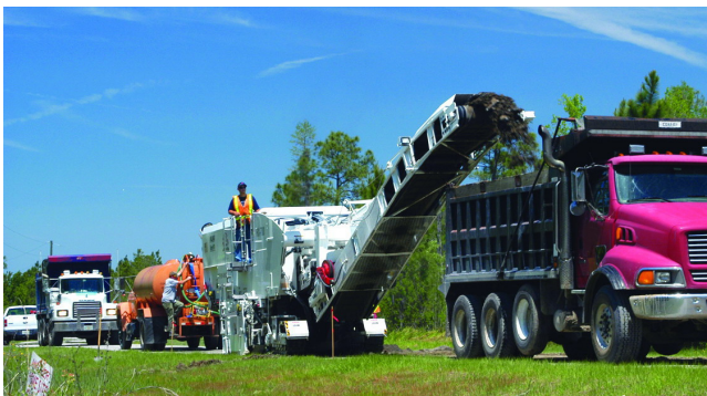
Figure 4. Asphalt is the most recycled construction product in the United States. The energy, emissions and environmental impact of recycling must be quantified. (Image courtesy of Asphalt Pavement Alliance)
